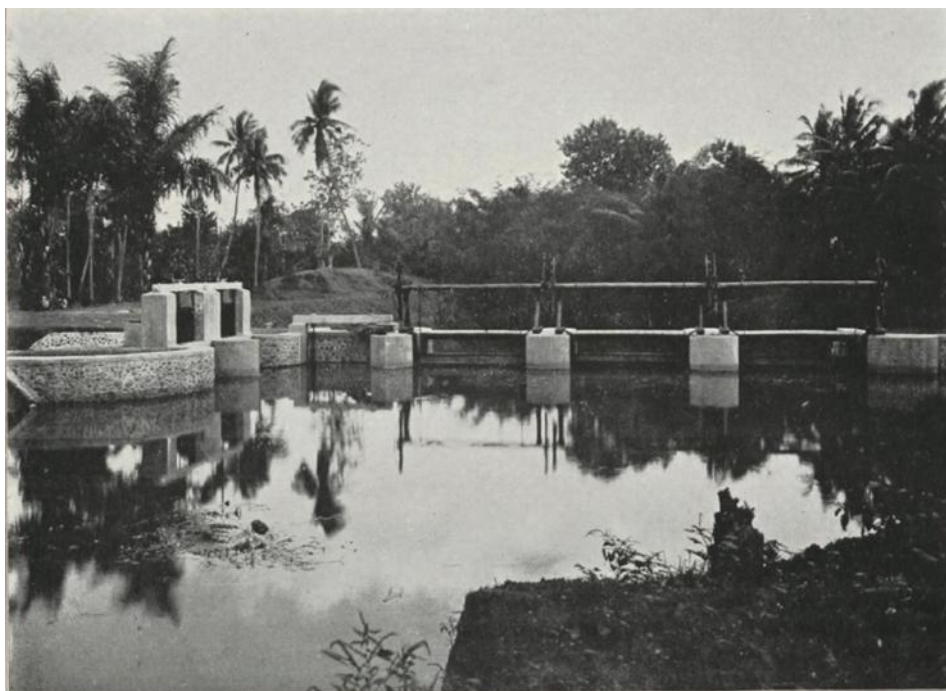
Figure 4. Modern irrigation system with concrete framework in Java, early 20th century (Numans, 1918).
