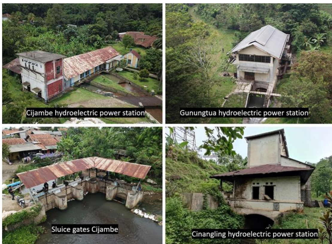
Figure 2. Photographs of the Cijambe, Gunung Tua, and Cinangling Hydroelectric Power Plants (Authors' Source).
