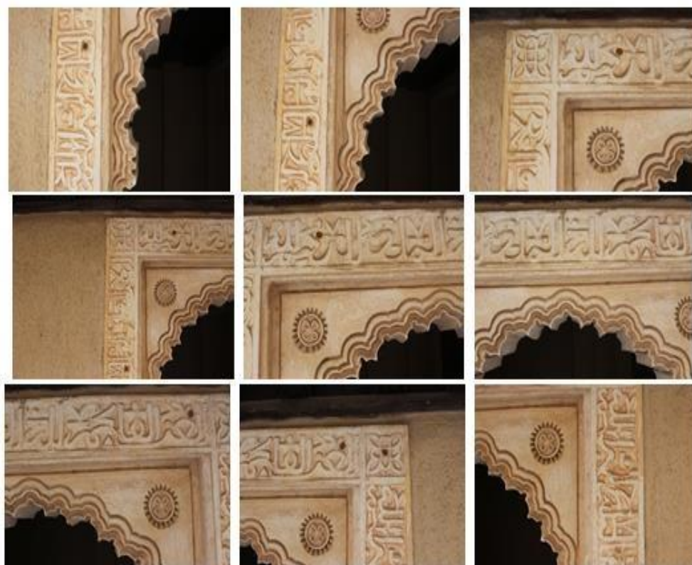
Figure 3. A series of corresponding images to digitize a surface (source: Authors).
