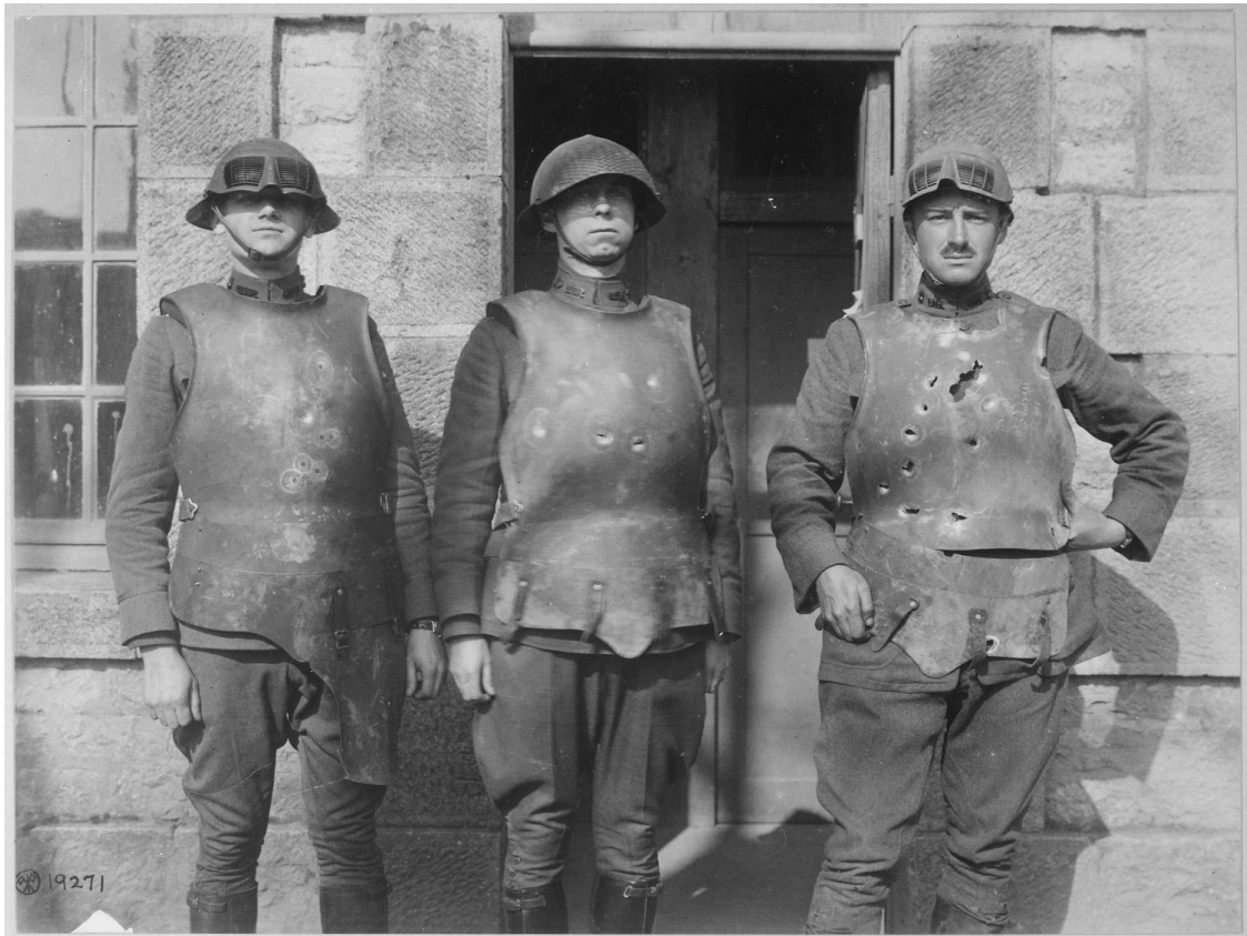
Figure 4. Result of Ordnance Department body armor test at Fort de la Peigney, Langres, France. Exhibit of body armor, heavy weight, showing effect of pistol, rifle and machine gun fire. (Army Ordnance Department, 1918).
