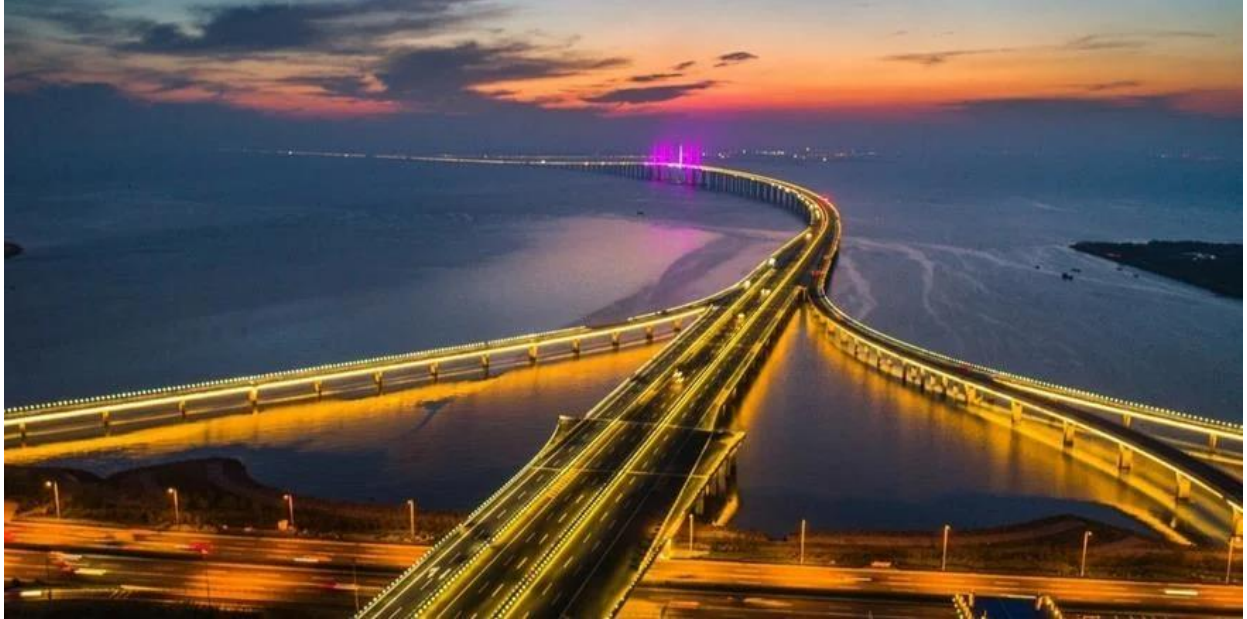
Figure 22. Danyang-Kunshan Viaduct (iXBT.com, n.d.).
