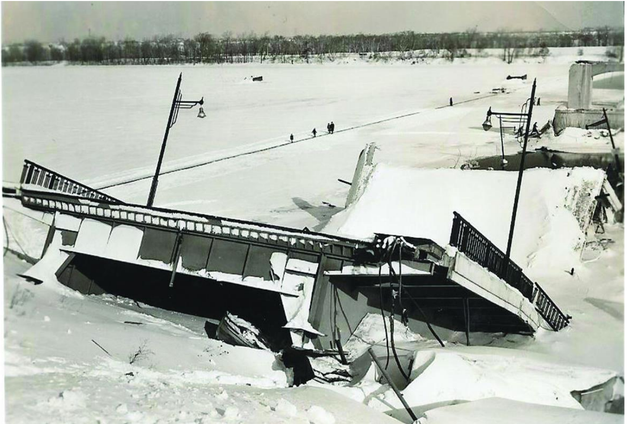
Figure 16. Duplessis bridge collapse (Lambie, 2021).
