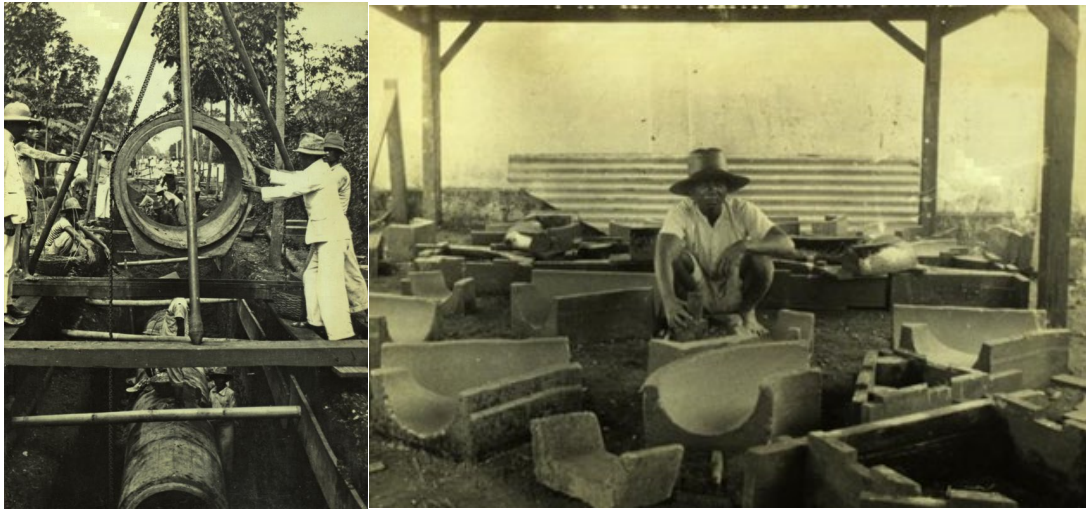
Figure 2. The installation of sewer pipes and the construction of concrete joints for sewerage in Bandung took place between 1929 and 1930 (KITLV 157009, KITLV 157013).
