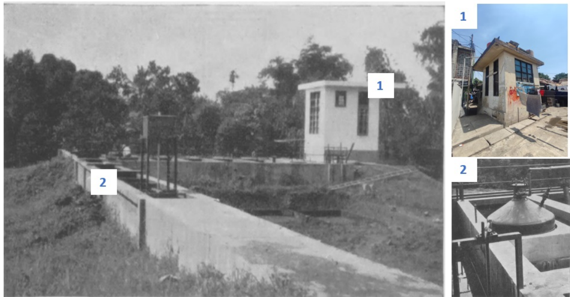
Figure 7. The sewage treatment plant, Imhoff Tank, in Tegallega, Bandung. Number 1 shows the laboratory room, and number 2 shows the methane gas collection tube (Mom, 1941, p. 163; personal documentation, 2023).
