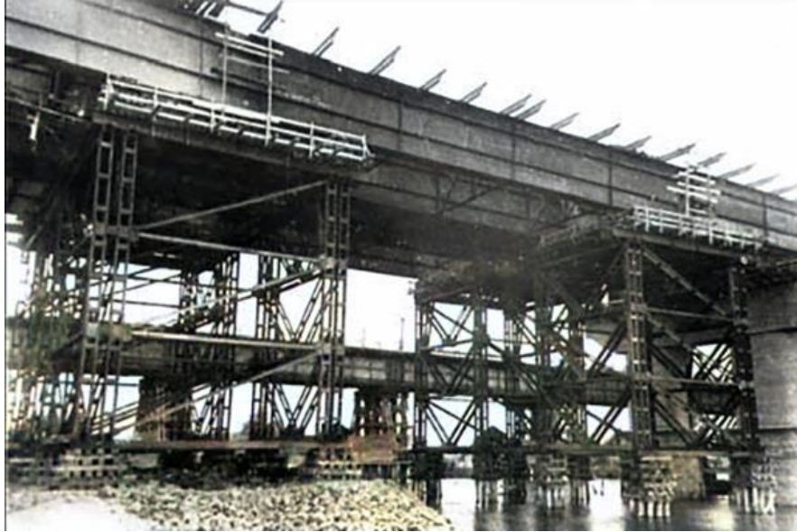
Figure 7. General view of welded site butt in the span (Lobanov & Kyrian, 2013).
