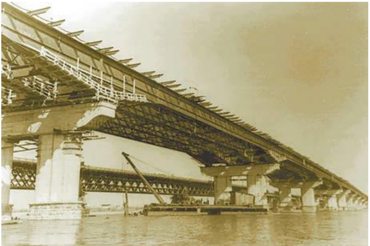
Figure 6. Construction of an all-welded bridge in Kyiv (Lobanov, 2020).
